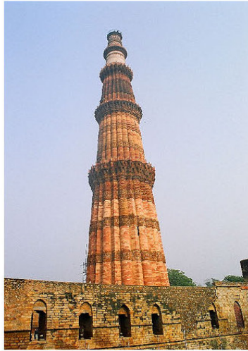
Fig. 4. Qutab Minar a 72.5 m tall minaret at Delhi. The upper two floors were dislodged during an earthquake in 1803. This was subsequently repaired.
